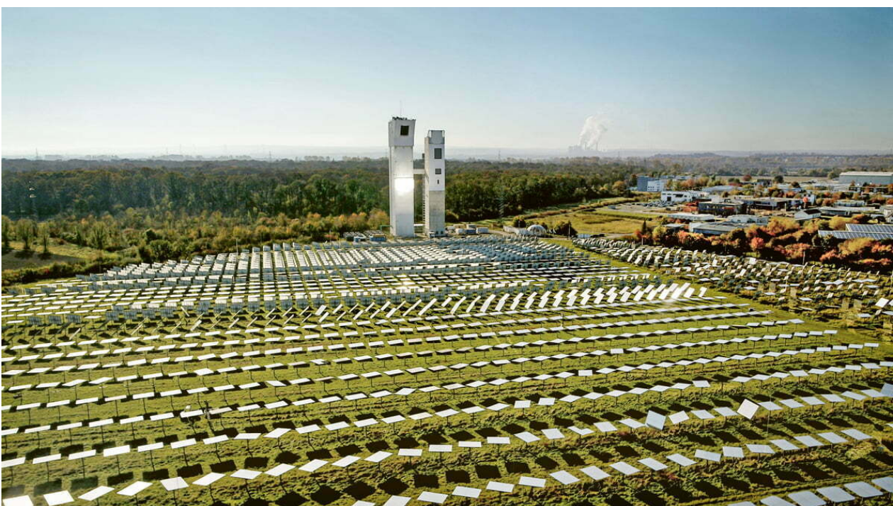
Test facility in the solar tower of the German Aerospace Center: the receiver in the tower absorbs the sun's rays reflected
