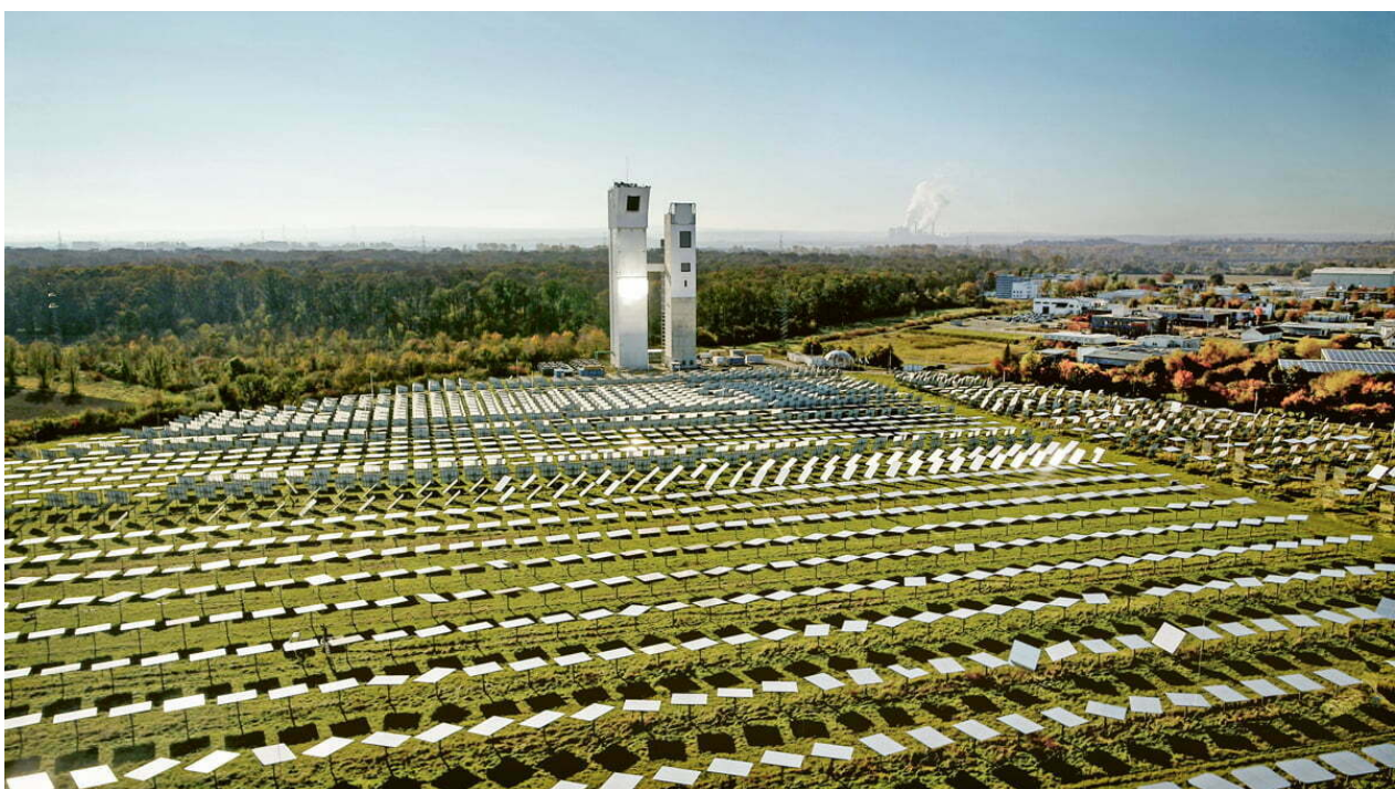
Test facility in the solar tower of the German Aerospace Center: the receiver in the tower absorbs the sun's rays reflected
