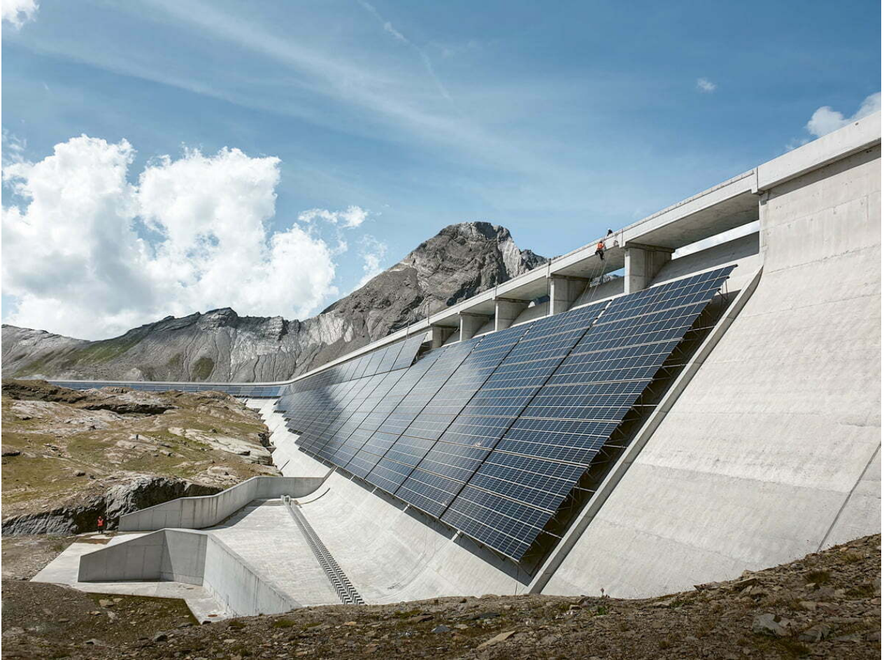
Switzerland's largest alpine solar plant on the Muttssee dam at 2500 metres.
