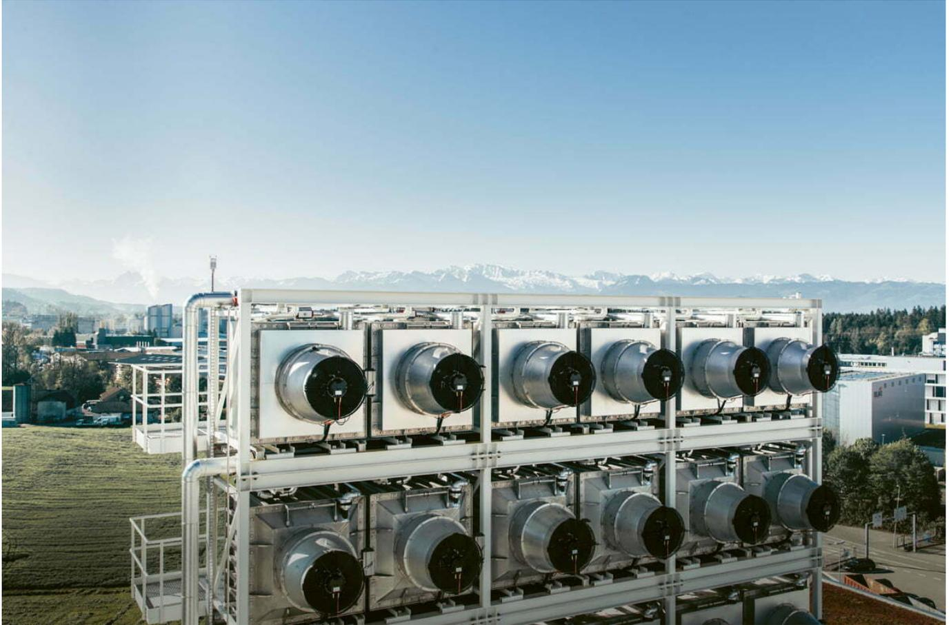
ETH spin-off Climeworks is a key player in the rapidly growing global market for the direct air capture process in which CO<sub>2</sub> is filtered out of the atmosphere and stored in the ground. The image shows a plant in Hinwil.
